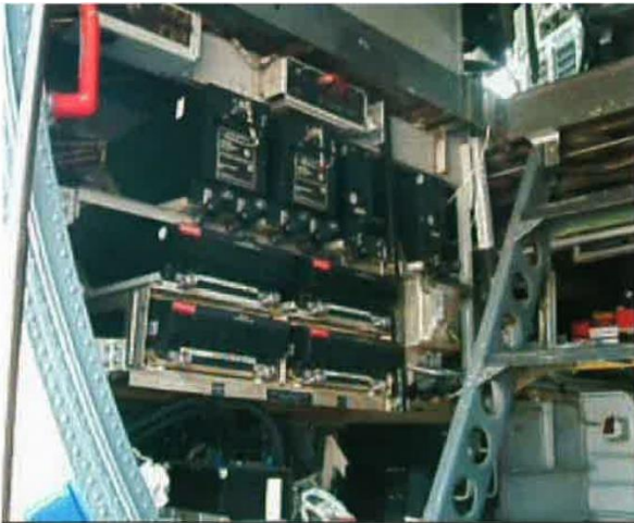
Under-Deck Avionics Shelf Installation
